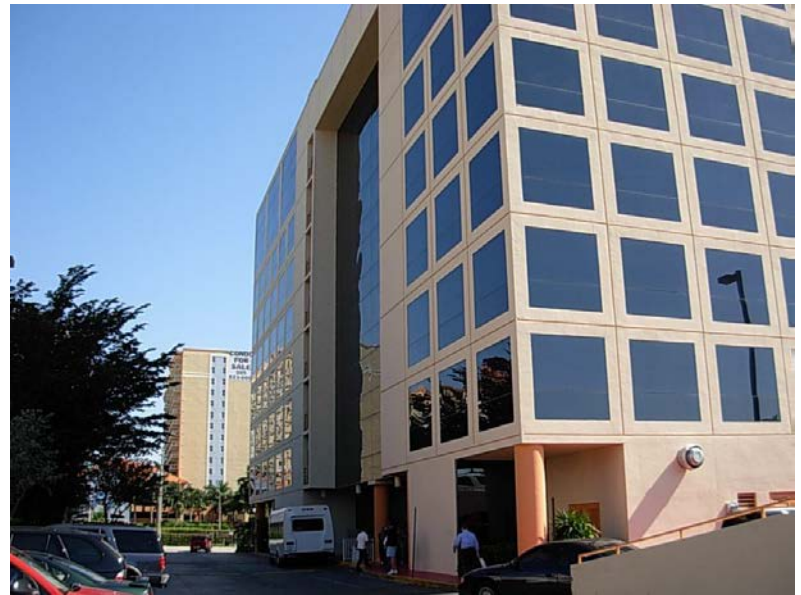
VIEW OF OFFICE ENTRANCE –FACING NORTHEAST
