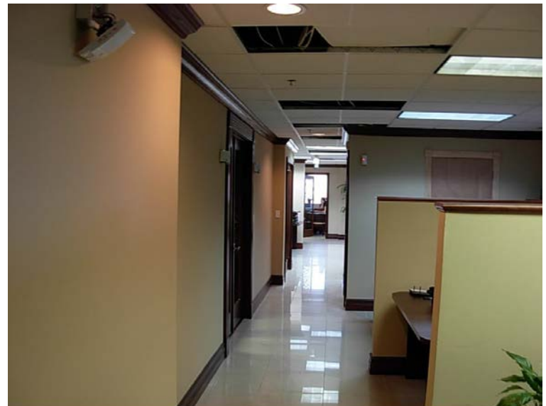
VIEW OF 9TH FLOOR OFFICE – EVIDENCE OF NEW SAFETY SYSTEM INSTALLATION
